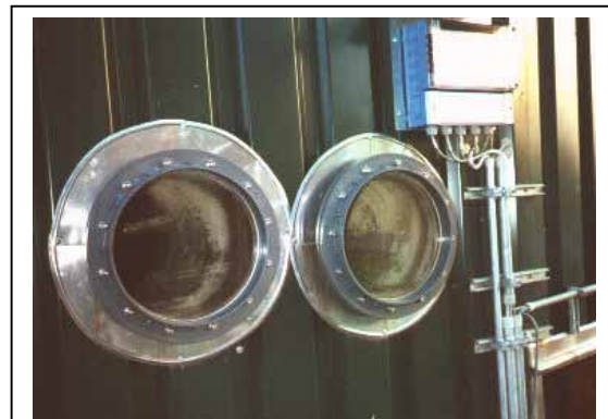
Figure 11: Control glasses for an industrial digester for solid organic waste, TBW, Germany
